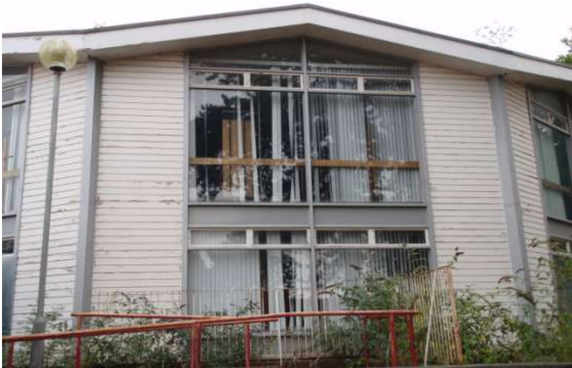
Plate 23. Close-up of one of the library panels set into a prefabricated steel frame (painted grey) and roofed with a lightweight polygon structure
