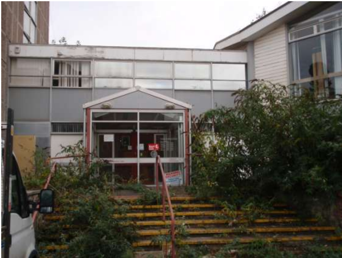
Plate 8. Entrance to the double storey corridor linking the admin block on the left and the reading room on the right. Modular construction with factory supplied external panels and a later porch
