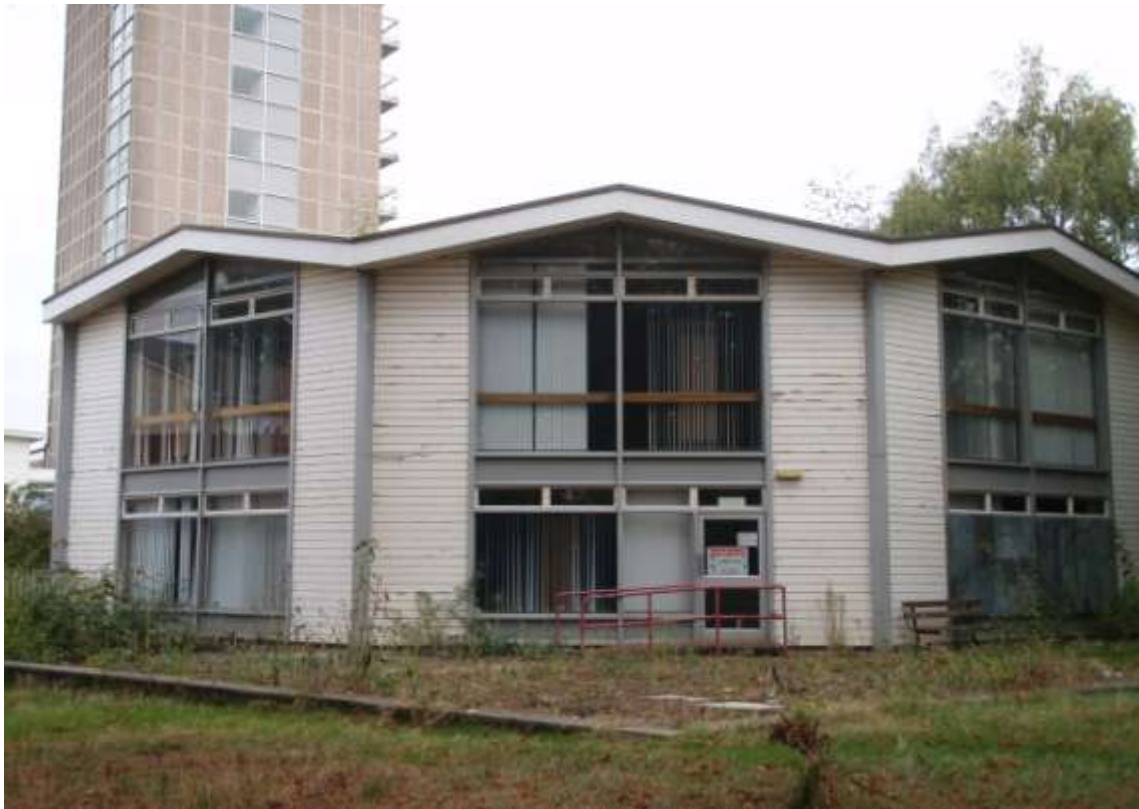
Plate 22. Exterior view of library showing modular panels
